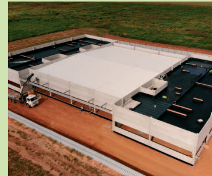
Works in progress of the physical-chemical and microbiological analysis laboratory
